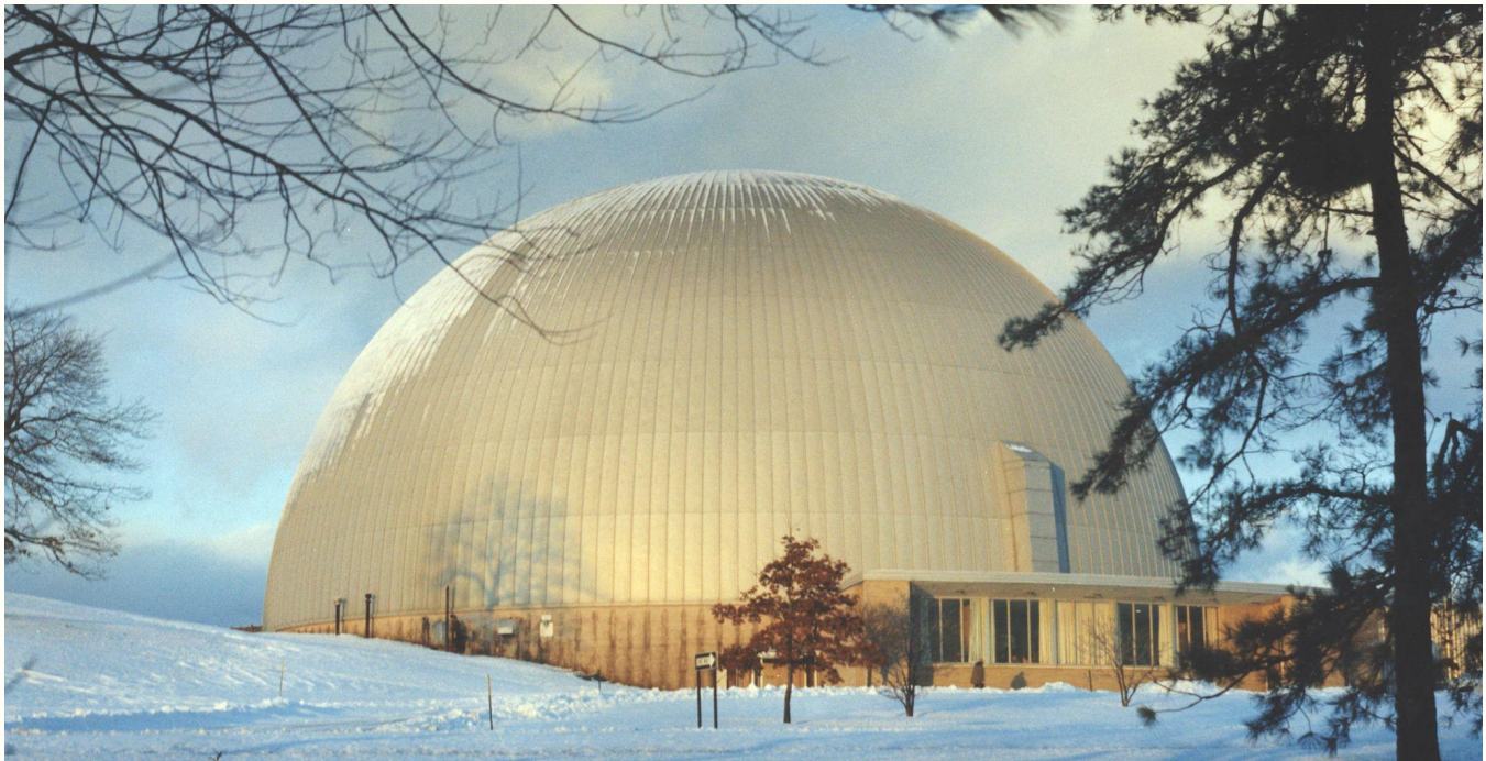
Containment dome for a test reactor at Brookhaven National Laboratory in New York (Photo from U.S. Department of Energy/Flickr)
